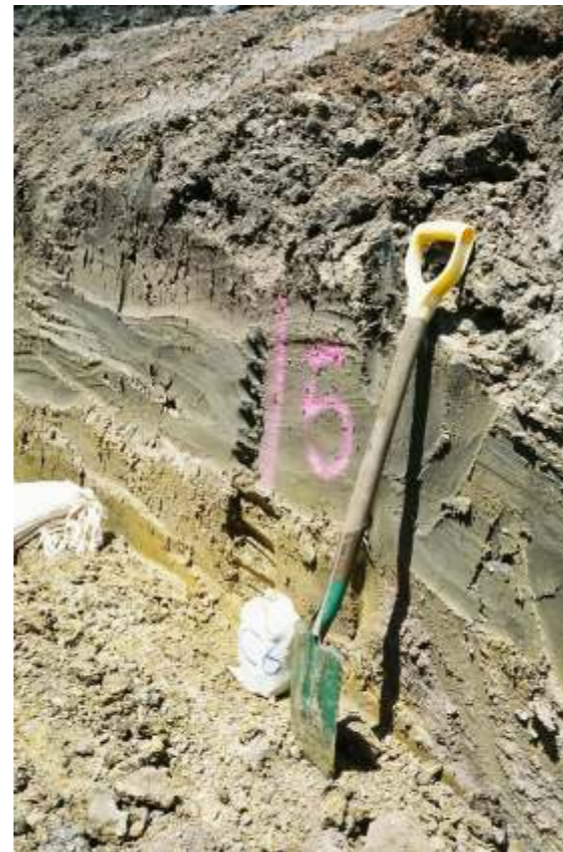
Photo - south side of trench, at 5 metres west of point "504" Sample # 6 i.e. B6 above C6 below - bedrock/basalt interface
